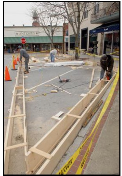
Travis Ponin of Pomfret, left, Mel Hawes of Plainfield and John Malarkey of Brooklyn work on concrete footing for a patio project Wednesday, March 26, 2008 on Main Street in Putnam. Photo by John Shishmanian.
